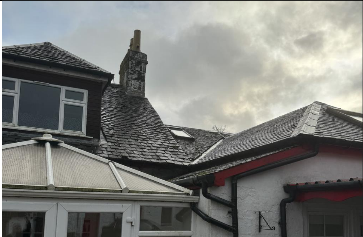
Figure 7 Images of external roof link between house and stables showing slate covering and metalworks
