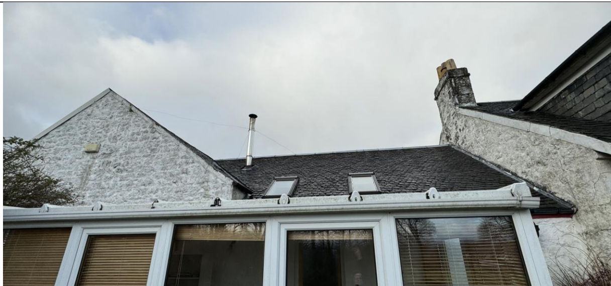
Figure 8 Images of external roof from rear showing slate covering, rooflights and metalworks
