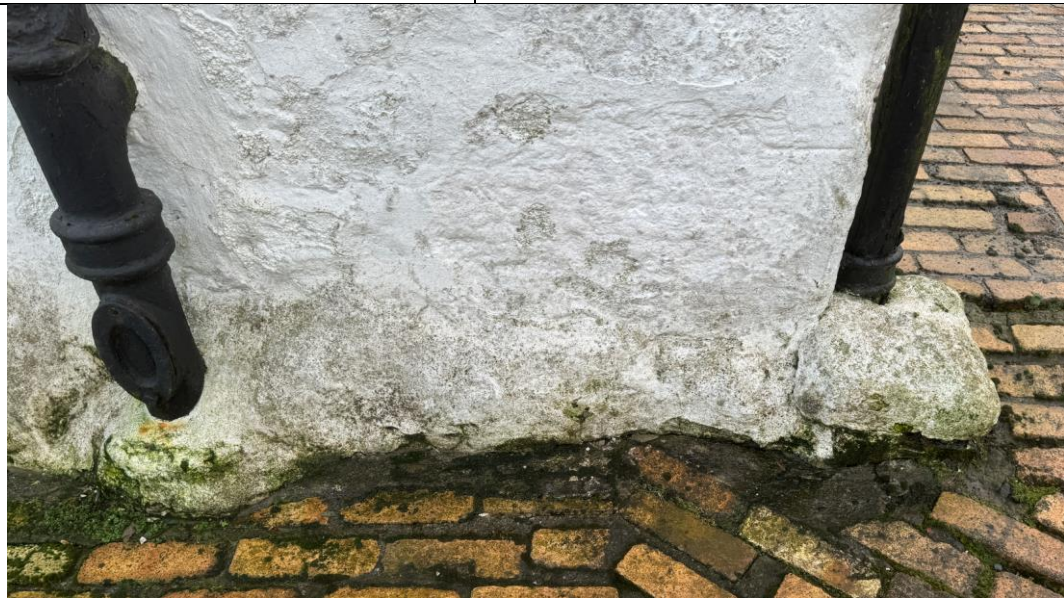
Figure 26 external gable wall with rocks in the wall build-up at the base
