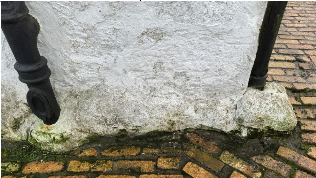
Figure 26 external gable wall with rocks in the wall build-up at the base
