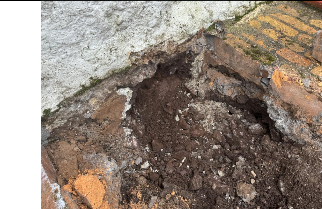
Figure 30 Image of the trial pit showing the existing build-up, ground condition and lack of any foundations
