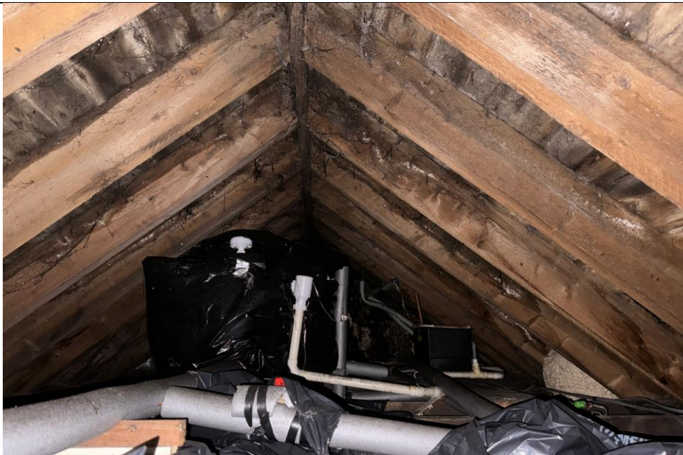
Figure 10 Inside main farm building roof space. Showing signs of water ingress and rot
