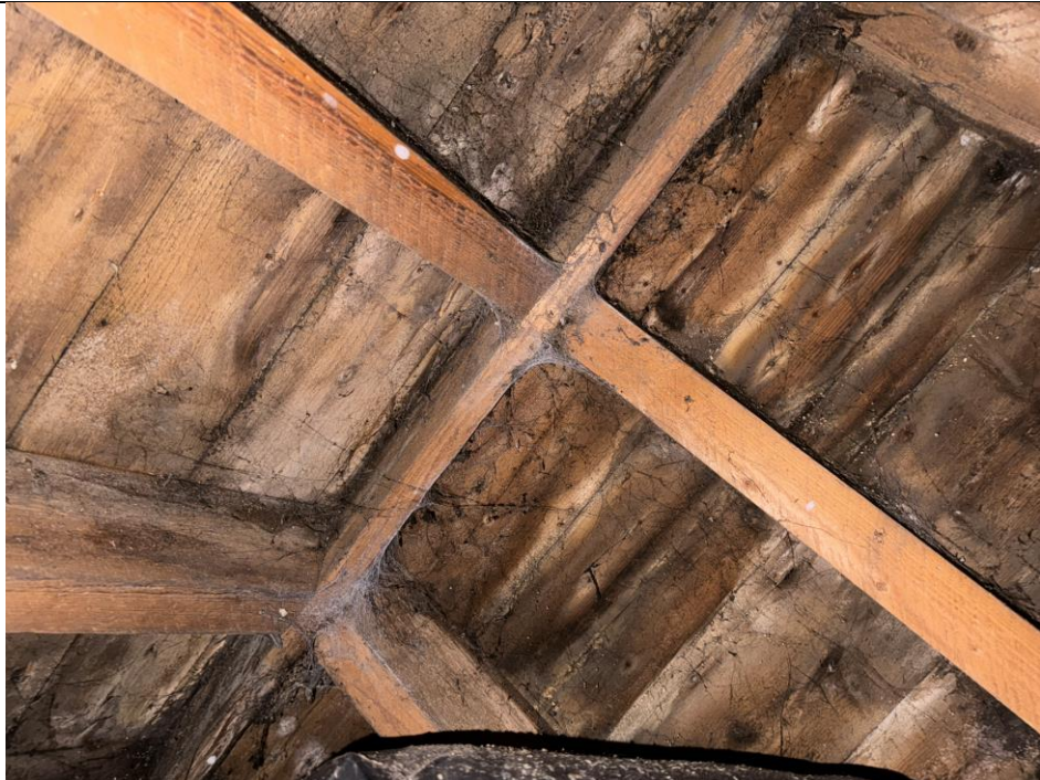
Figure 9 Inside main farm building roof space. Showing signs of water ingress and rot
