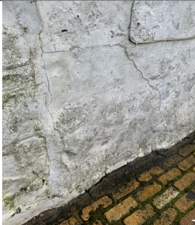
Figure 25 External gable wall showing evidence of minor cracking to the external finishes.
