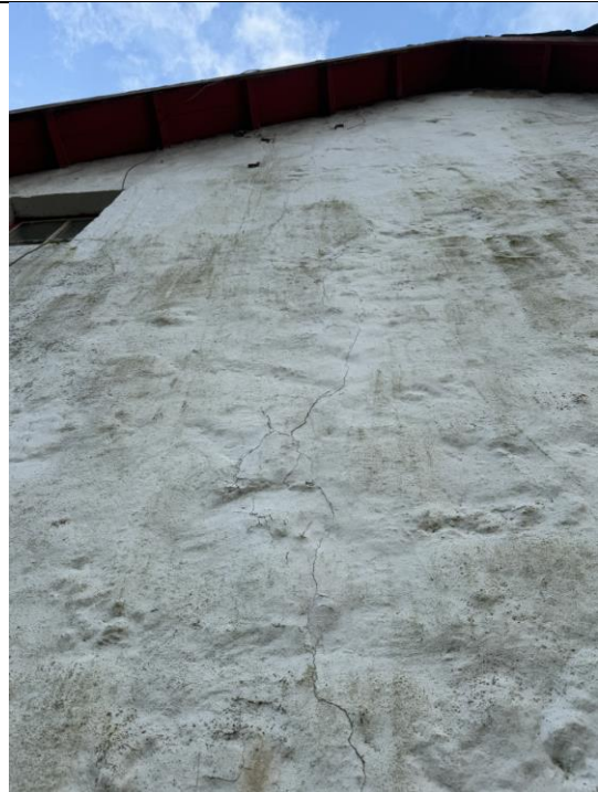
Figure 24 External gable wall showing evidence of minor cracking to the external finishes.
